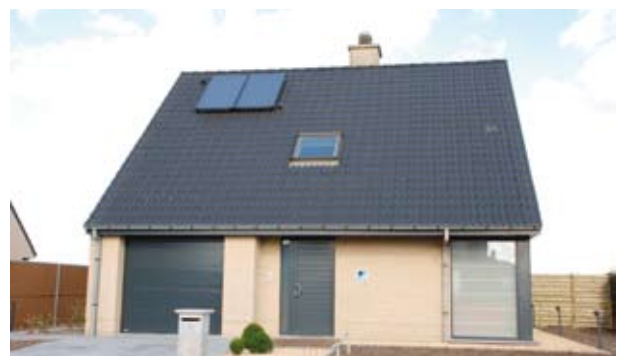
➔ Solar collectors are combined with the heat pump system to provide domestic hot water for the Daikin Energy Saving House
